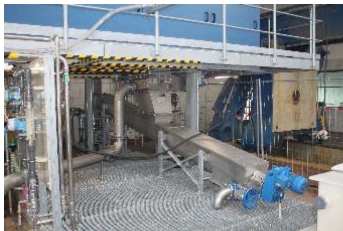
The inclined conveyor moves sludge from the top into the silo.
