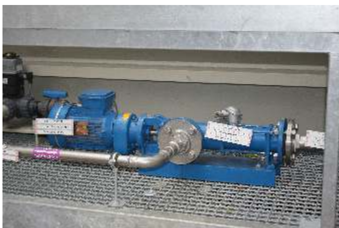
Allweiler® progressive cavity pump used as metering pump.
