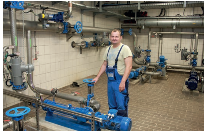
Even after twelve months of continuous operation, the Allweiler Optifix progressing cavity pump of the AEB1F series from CIRCOR shows no sign of wear, according to the experience of Marcel Fricke, Technician at the sewage plant Rollsdorf.
