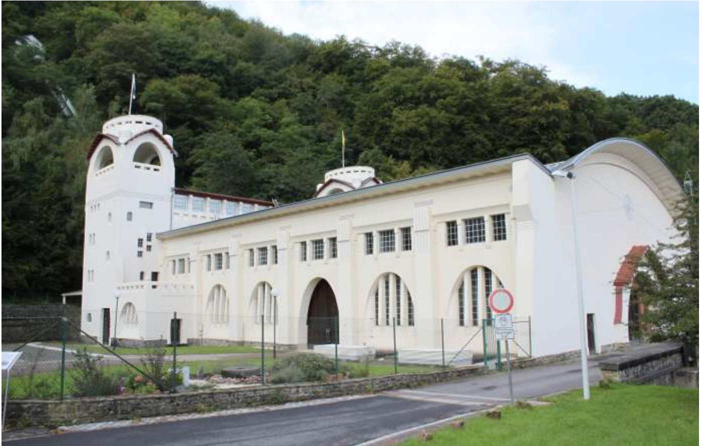
Heimbach is Germany's most beautiful Art Nouveau power plant and is kept in its original condition.
